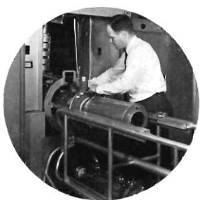
FIG. 12. Roll new tube into magnetics.
