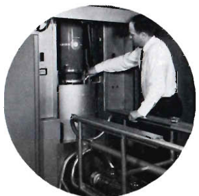
FIG. 8. Disconnect water-inlet hose.
