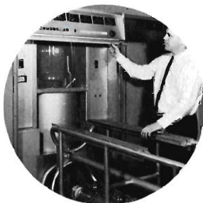
FIG. 6. Lift meter panel.
